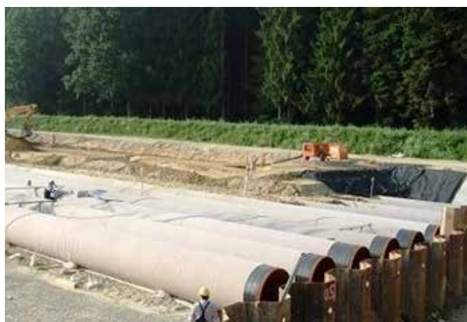
Laying of pipe strings for natural gas storage [1]
